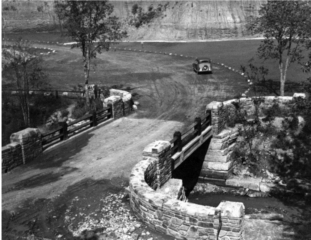
Quarry Picnic Area Bridge built by CCC, Euclid Creek Reservation 1935 (Cleveland State University Library Special Collection)
