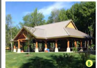
LARGE RESERVE SHELTER
