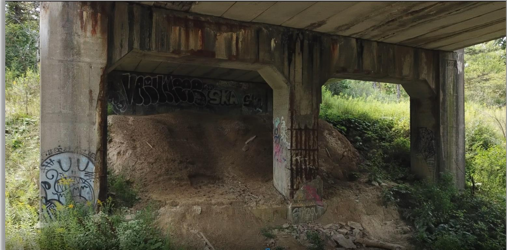
Hawthorn Bridge Infrastructure, South Chagrin Reservation, Photo Credit: India Johnson
