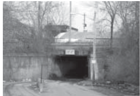
Booth Avenue Bridge
