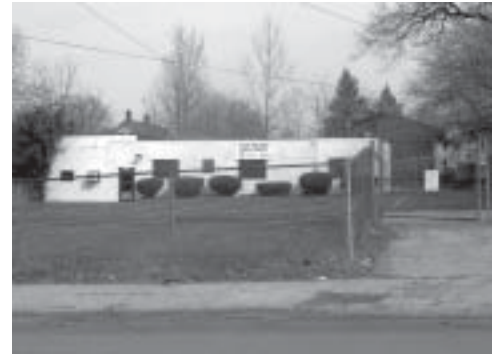
St. Luke's Church with parking, Union Avenue
