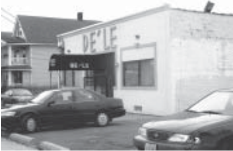
Commercial property with recent storefront and signage improvements
