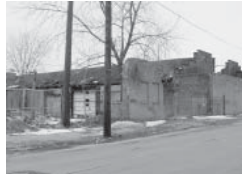
Deteriorated industrial property on East 91st Street
