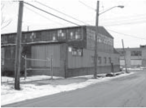
Commercial Forge, East 93rd Street
