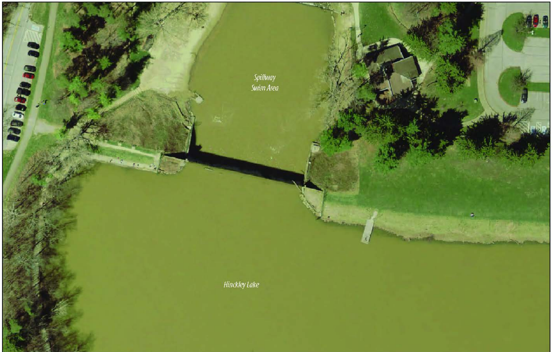
Hinckley Reservation Existing Conditions: Dam and Spillway
