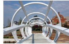
NEW PEDESTRIAN BRIDGE
