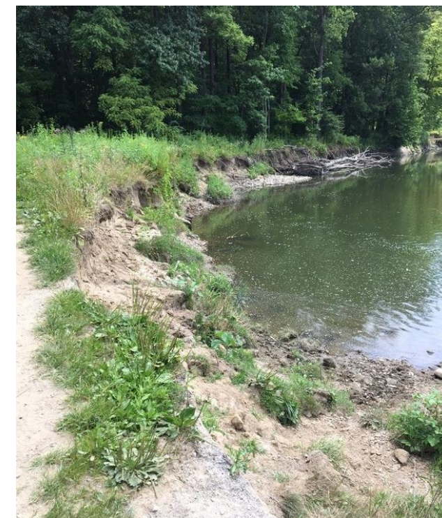
Eroding streambank on Chagrin River
